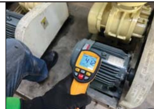
Photo#13 : Check the temperature of the motor.
