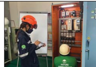
Photo#15 : Check the Air Blower's current & condition.
