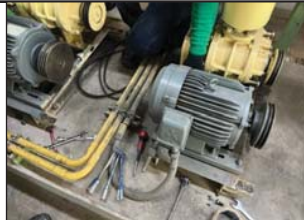
Photo#2 : Demolish the work & inspect the Air Blower.
