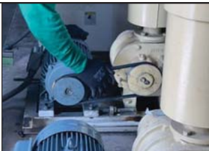
Photo#8 : Replacing the v-belt of the Air Blower.
