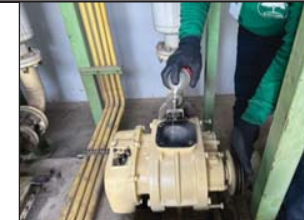
Photo#10 : Spray rust remover to prepare the blower.
