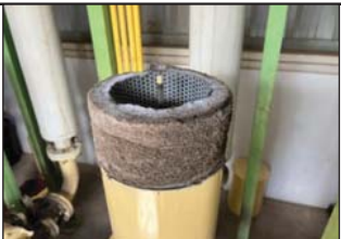
Photo#5 : Before replacing the air filter in the Air Blower.
