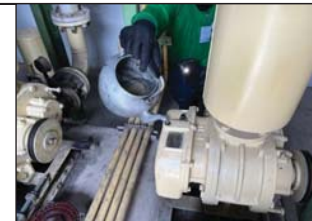
Photo#11 : Changing the oil & grease in the Air Blower.
